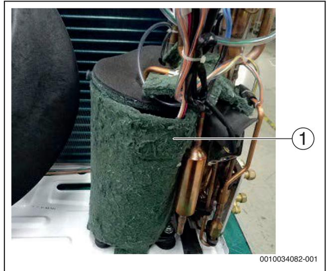
Fig. 108 Removing compressor cover 1
