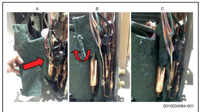
Fig. 110 Removing assemble cover
